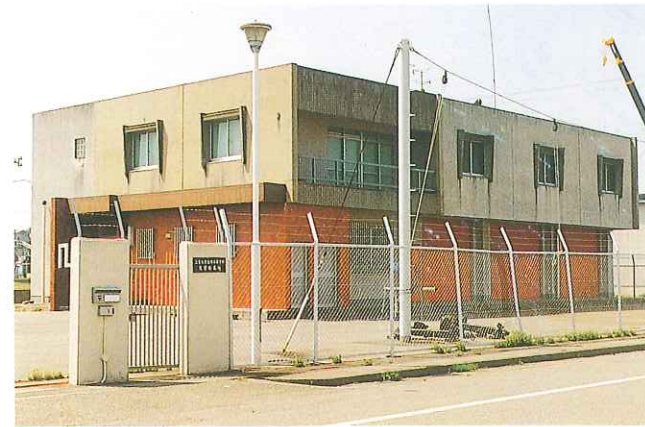
▲船具保管庫 OFFICE & WAREHOUSE
