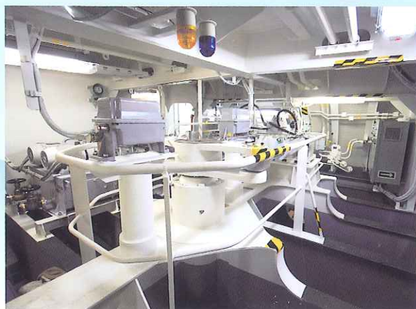
舵取機室 / Steering engine room
