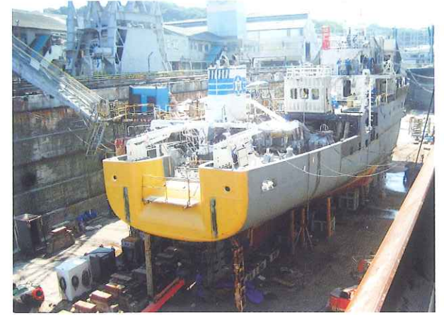
煙突搭載 / Installation of funnel
